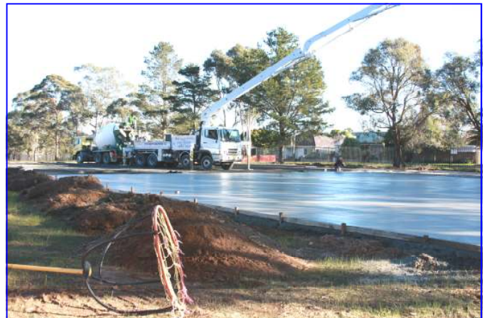
The new concrete slab being laid for our new sports courts.
